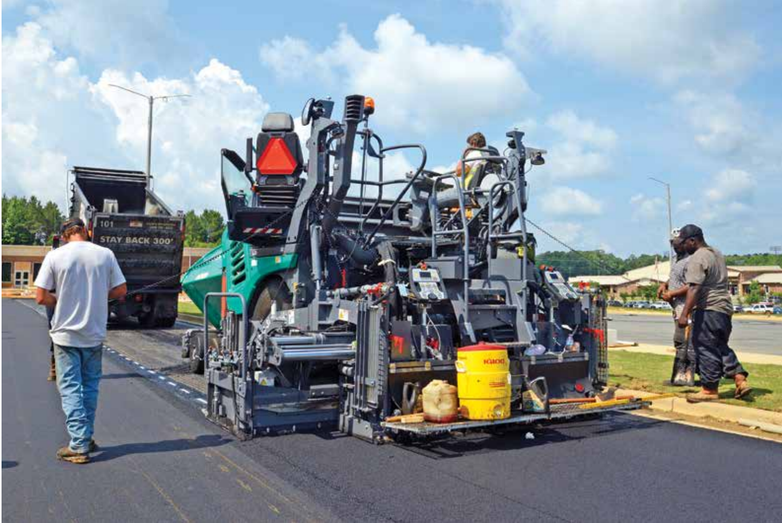
ST Bunn Construction Company pairs its VÖGELE Super 1703-3i paver with a VF 500 front-mounted screed on a school parking lot in Buhl, Ala. Here, crews used the wheeled paver to place asphalt on a base course within tight radii around curves and parking lot curbs.
