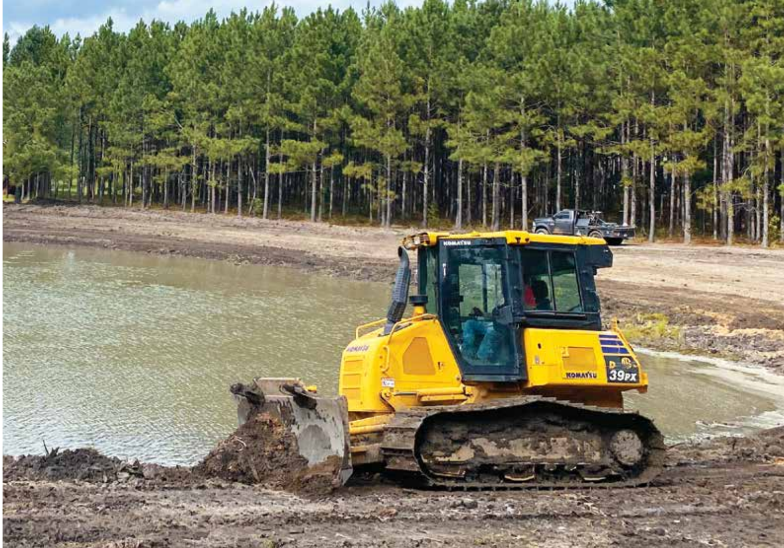
Triple B Land Services owner Ethan Bragg uses a Komatsu D39PX-24 dozer to fix the grade leading up to a pond's edge. "The D39 has great power for its size," noted Bragg. "Its ground pressure ratio allows it to float over wet material without getting stuck. It also has the slant-nose design that allows you to see the blade for fine grading."
