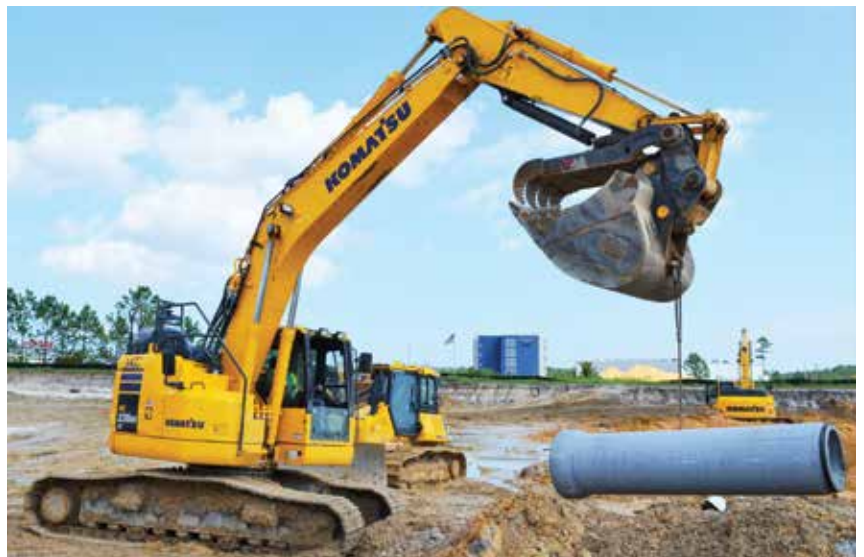
An operator places pipe with a Komatsu PC238USLC midsize excavator.
