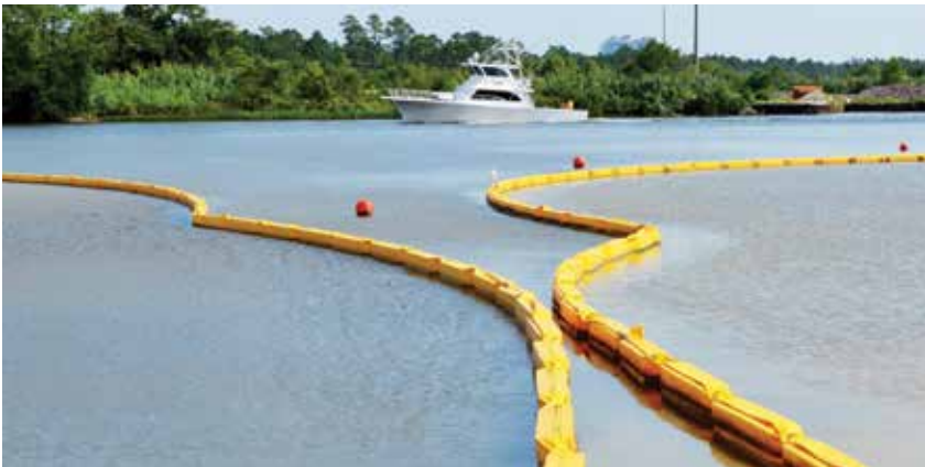
Turbidity curtains were placed before excavation began to ensure an environmentally friendly job site is maintained.
