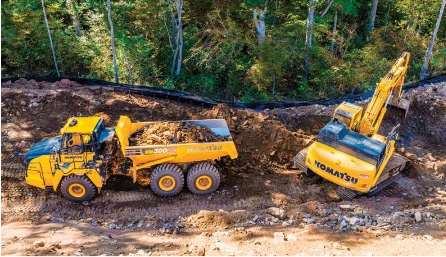
At Dogwood Site Contractors' Hickory Level job site, an operator uses a Komatsu PC490LC excavator to load material into the bed of a Komatsu HM300 articulated truck.
