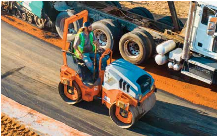
With a HAMM HD12 tandem roller, an operator compacts an asphalt mat.
