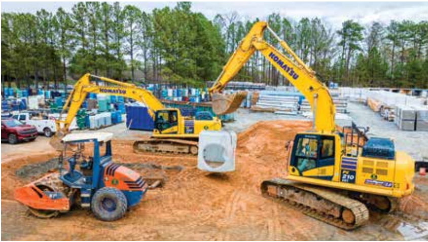
An operator moves part of the storm drain system into place with a Komatsu PC210LCi-11 IMC excavator, while another operator removes material from the ditch with a Komatsu PC360LCi-11 IMC excavator. CBH Contracting's fleet also includes a HAMM H7i compactor.
