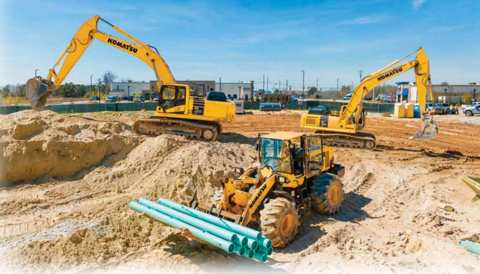
An operator transports pipe with a Komatsu WA320 wheel loader while a pair of operators use Komatsu PC360LC excavators to backfill recently laid pipe. "The two operators who sit in the loaders all day love them," said MSS President Daniel McCoy.
