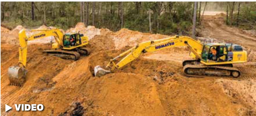
Operators work in tandem to remove bulk amounts of material with a Komatsu PC360LC excavator, then follow up and cut to grade with a Komatsu PC290LCi-11 IMC 2.0 excavator.
